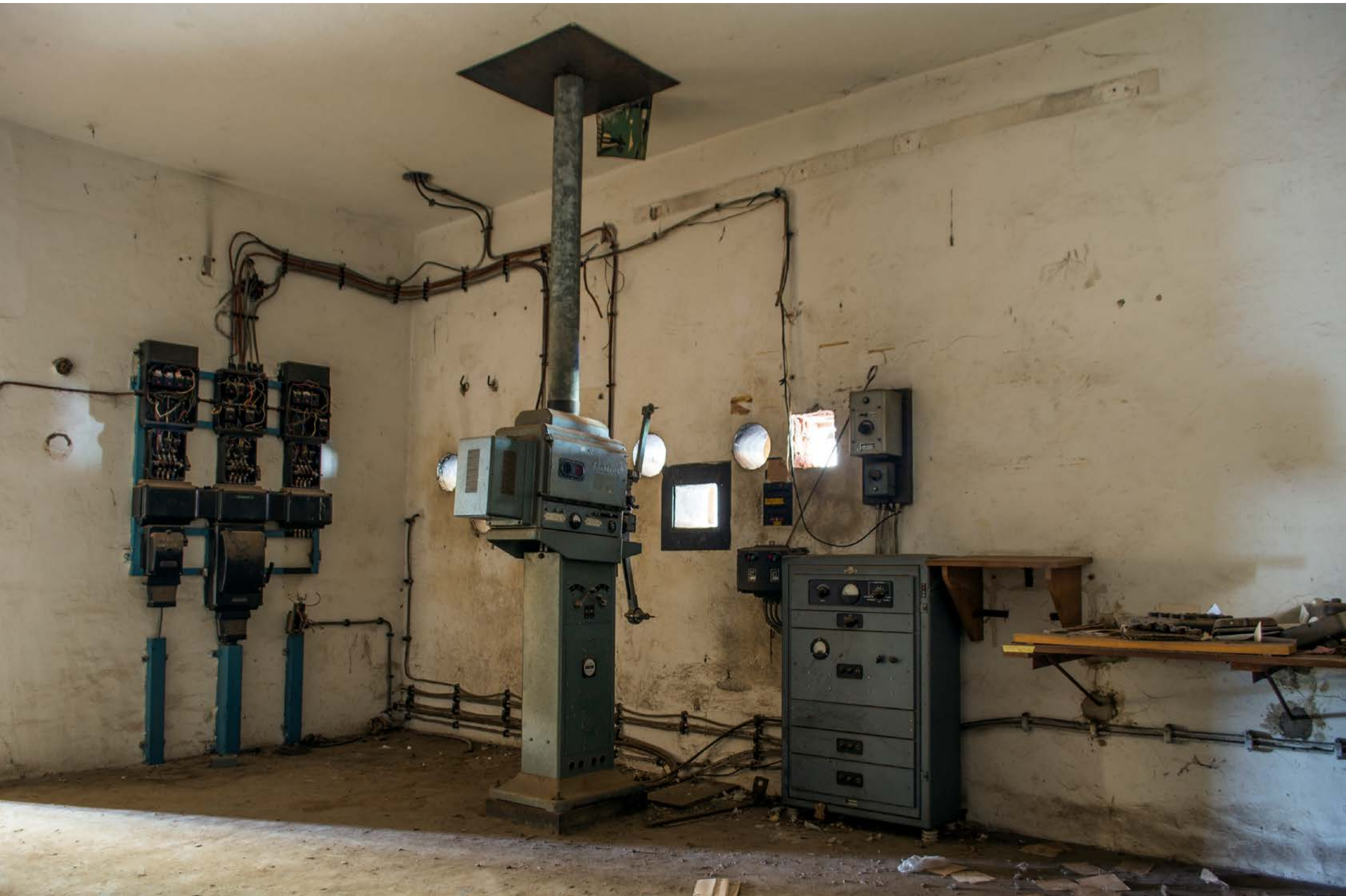
©Georges Senga, from the series Format. (Photograph taken in CLP, Likasi, in the south of DRC. CLP is owned by a large mining company, GECAMINE, that played a complicated role in the area, building libraries, swimming pools and cinemas in DRC.)
